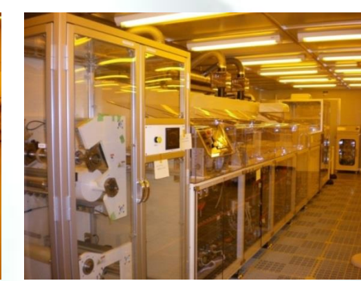
Wet clearing (FEBACS)
